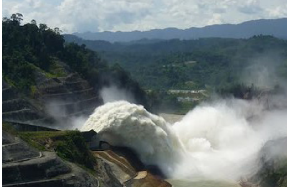
Photograph of a dam in Nepal
